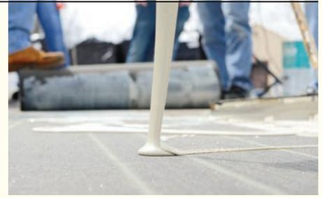
*Above: POWERply Endure BIO Adhesive TF is a bio-based roof membrane adhesive that's virtually odor-free.*
