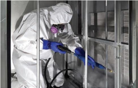
*Pure Air Control Services addresses indoor air-quality concerns through environmental consulting, building diagnostics, laboratory services and HVAC system hygienic cleaning and restoration. Above, an associate disinfects an HVAC system with high-temperature steam to restore airflow and energy efficiency while also improving air quality.*
